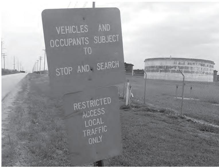
Oil storage tanks in Cushing, Oklahoma
