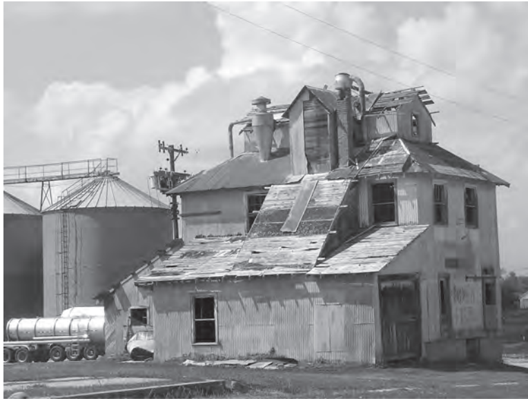
Former granary near Keystone XL route in Western, Nebraska
