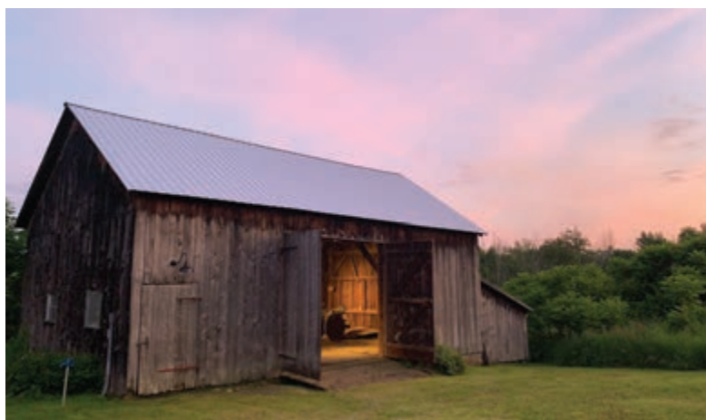
4. The Robert Frost Stone House Museum's newly restored historic barn
